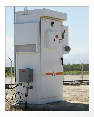
The CVD Series Drive includes all required automation equipment, eliminating the need for external PLC. It links directly with your field signals and is fully compatible with Well Optix, our remote monitoring system as well as other systems. Everything is assembled and tested before it ships to the field, so you have no need for additional installation and start-up expenses with multiple vendors.
